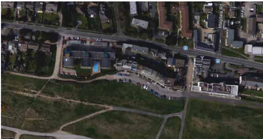
Aerial view of Ward Court (left) and Norfolk Crescent (right)
