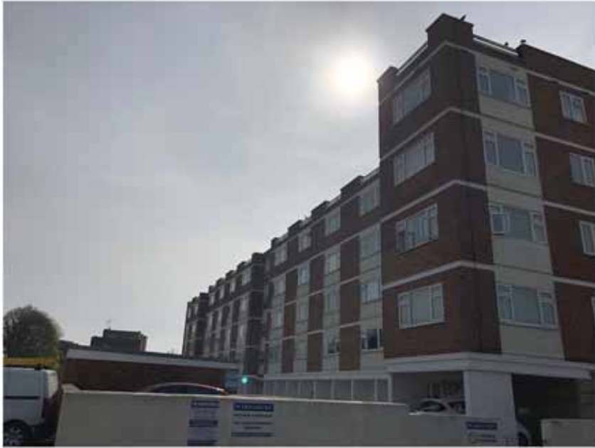
Plate 1 Ward Court, west end of building looking northeast
