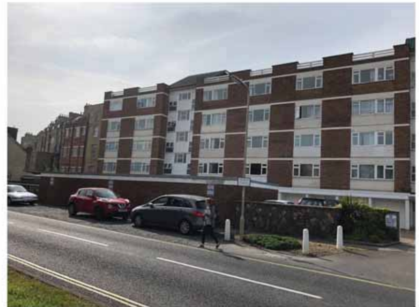
Plate 4 Ward Court and Norfolk Crescent, front north-facing elevation from Sea Front
