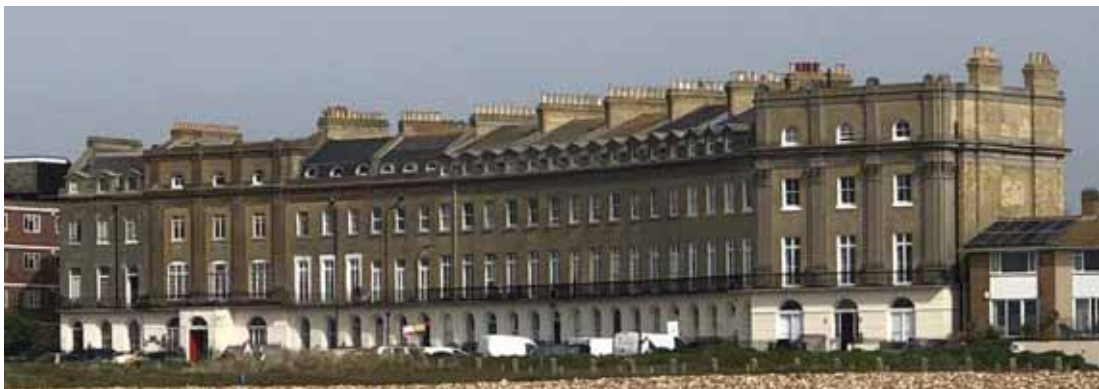
Norfolk Terrace, south-facing elevation
