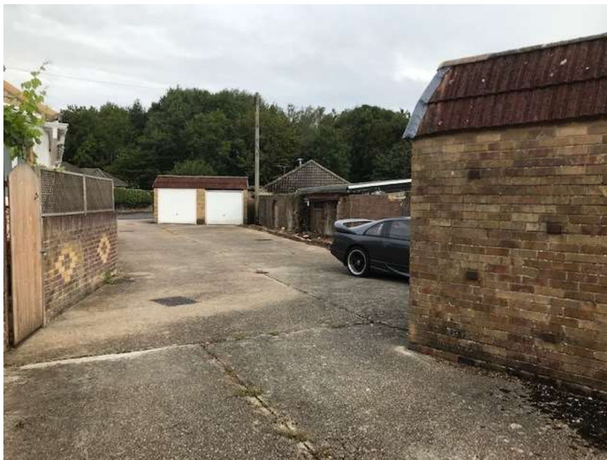
Fig.11 – Photograph taken from within the site looking north-west towards the end of garage Block B and hard standing area in front of garage Block A (foreground).
