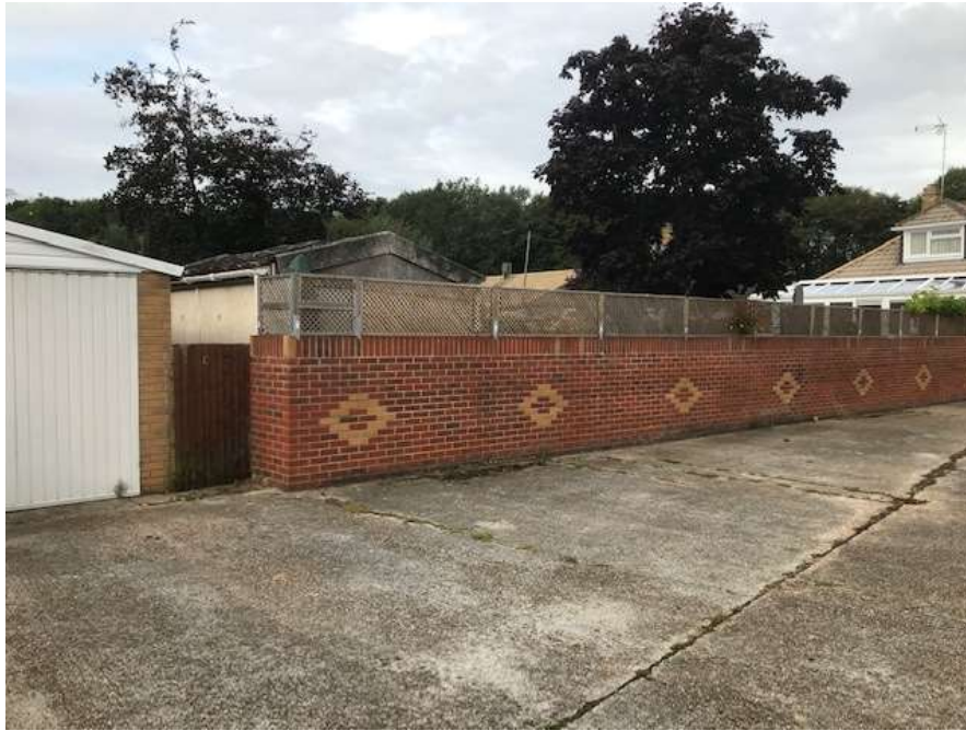
Fig.10 – Photograph taken from within the site looking west towards the brick boundary wall to 8 Willowdene Close and detached single garage (left).
