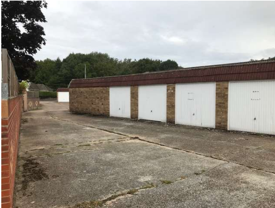
Fig.6 – Photograph taken from within the site looking north towards Block A with the hard-standing area in the foreground.
