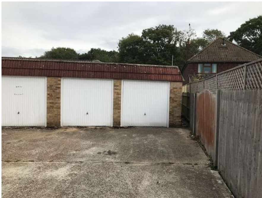
Fig.7 – Photograph taken from within the site looking north-east towards the end of garage Block A and the boundary fence to the rear garden of 115 Hulbert Road (right).
