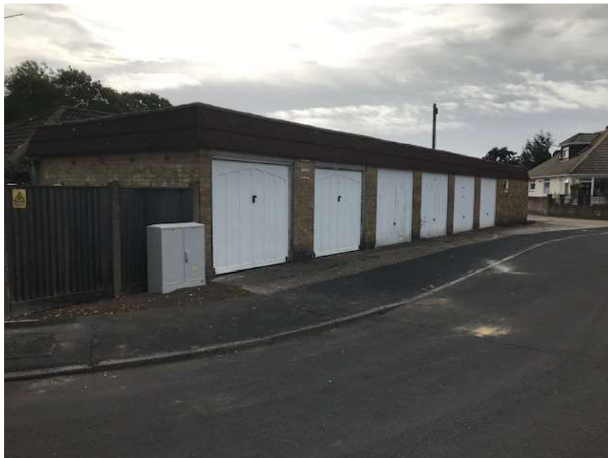
Fig.1 – Photograph taken from Willowdene Close looking south towards the front elevation of garage Block B.
