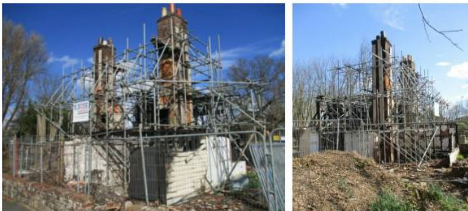
Figure 4 & 5 : Structural Scaffolding (March 2019)
