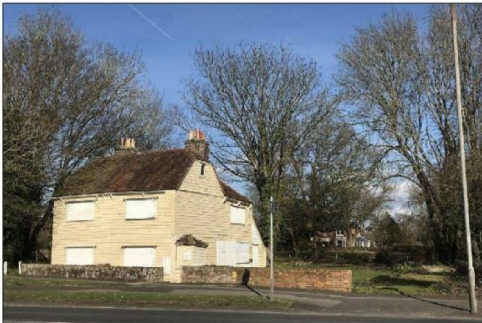
Figure 20: 59 & 61 Langstone Road. Vacant with boarded up windows. (The News, 2019)
