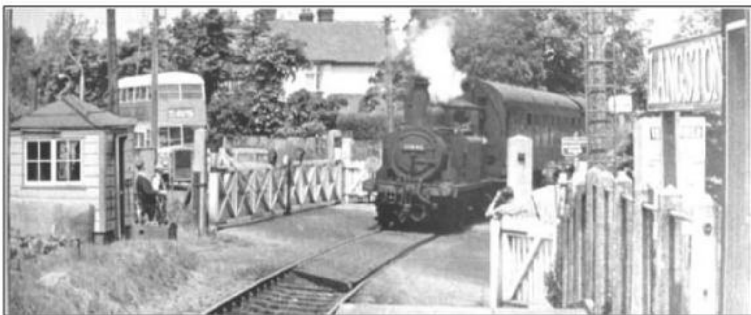
Figure 16: Langstone Level Crossing (Griffiths, G, n.d)
