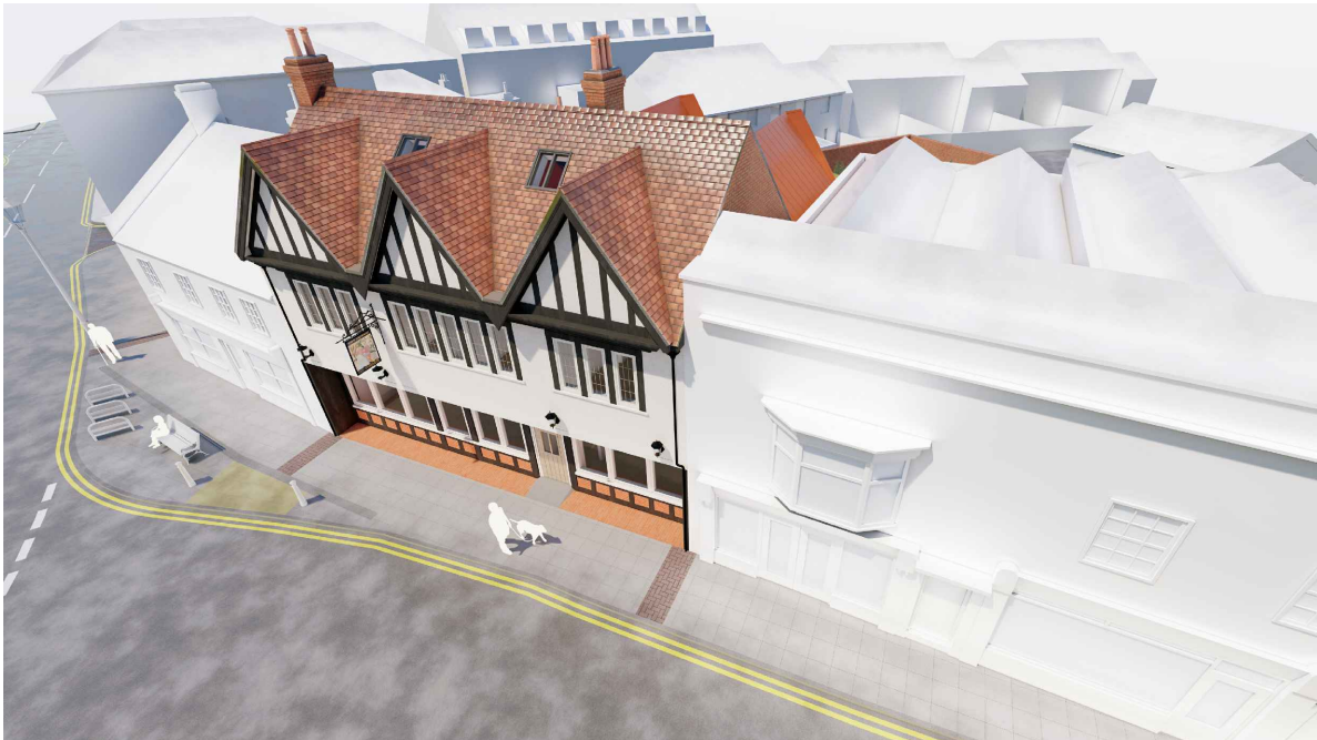
aerial view from west street
