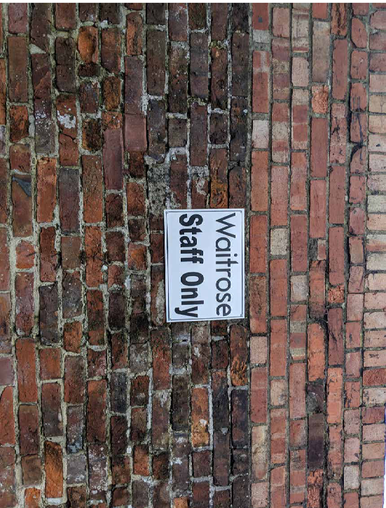
Current signage in-situ/Proposed signage location
