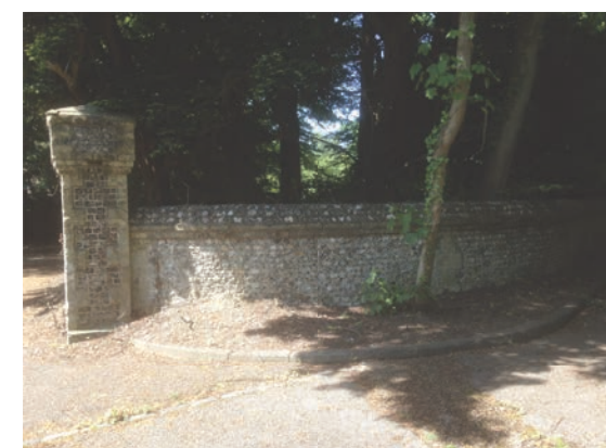
Remnant estate boundary wall and entrance pillar. Missing pillar will be represented with new clipped yew pillar in estimated location of original pillar as part of Lodge curtilage
