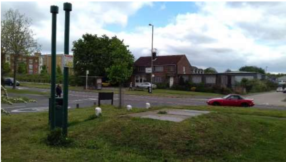
Figure 2. Gas Structure on Corner of Dunsbury Way and Bramdean Drive.
