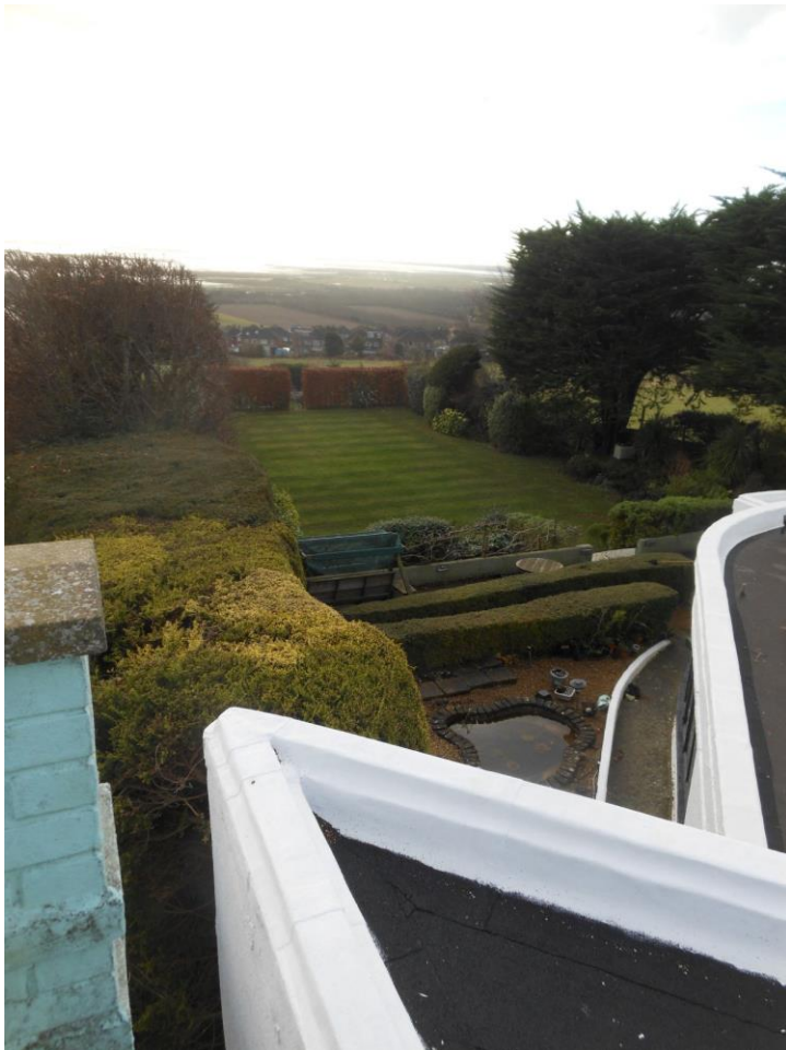
Junction of west elevation with Sunspan house
