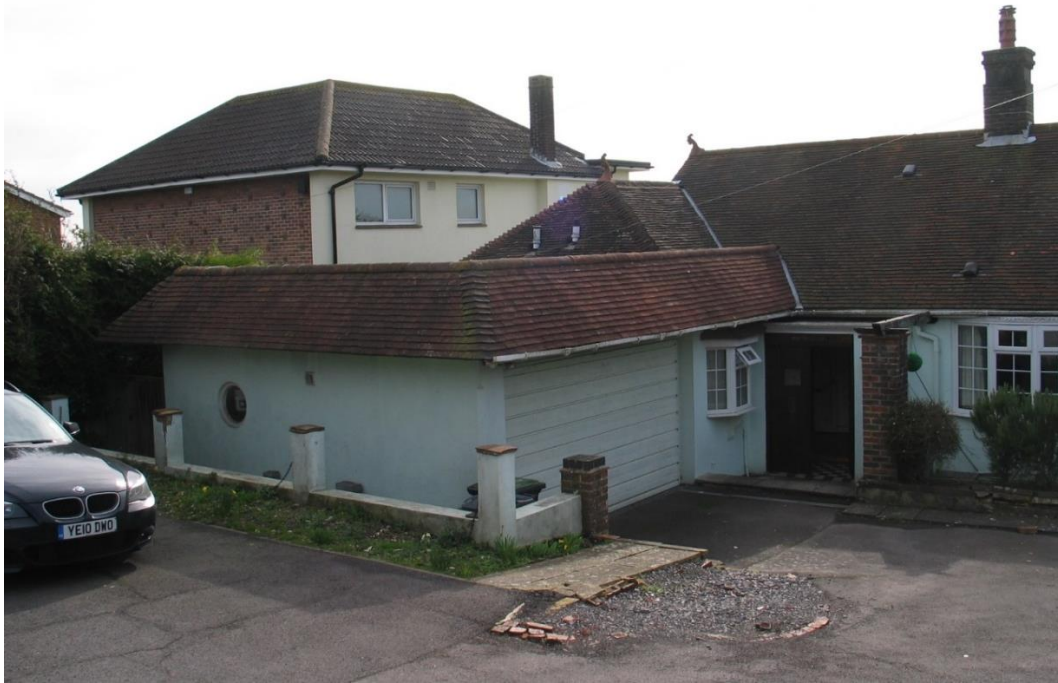
Part of north elevation showing existing garages
