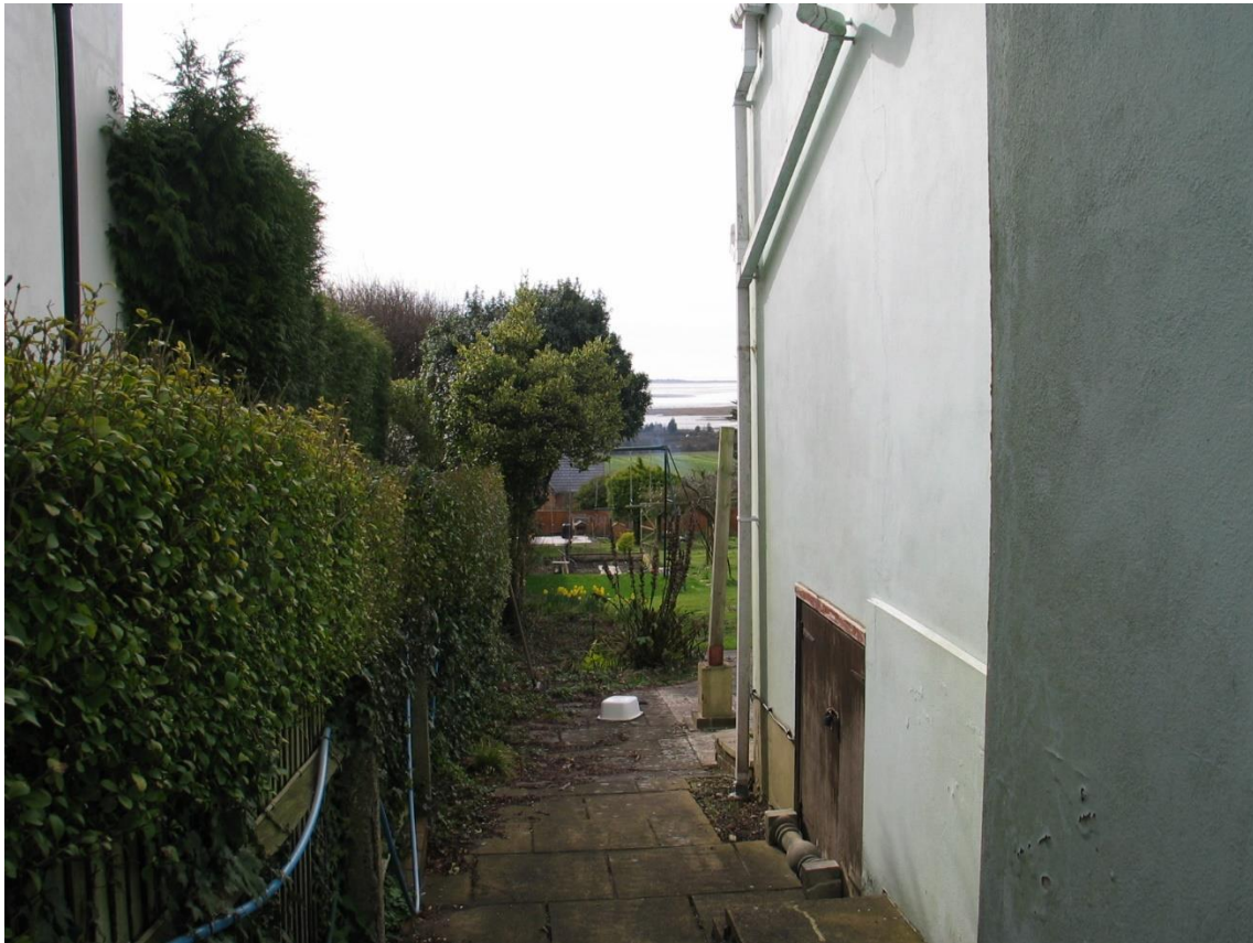
Part of east elevation looking south
