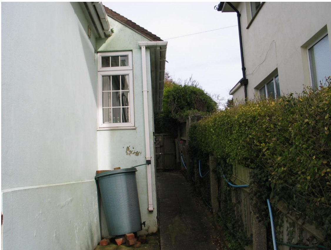
Part of east elevation looking north
