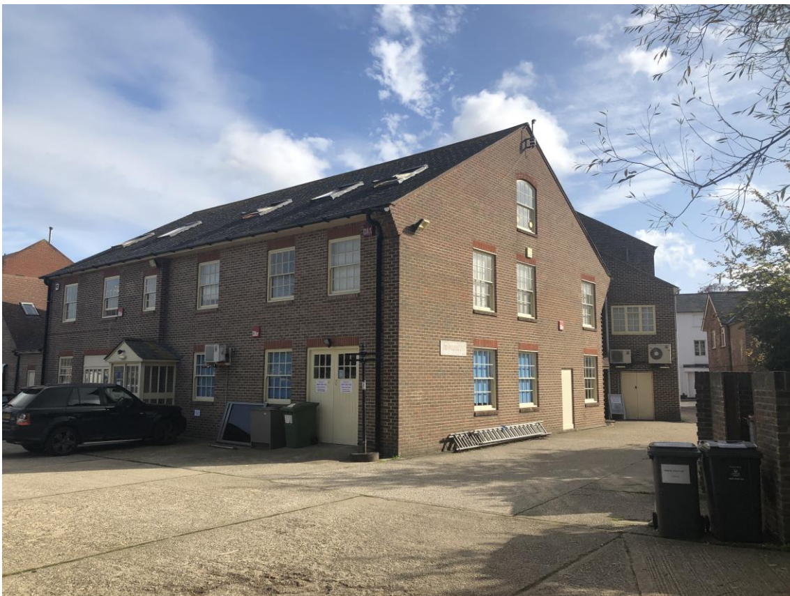
Figure 1: View of Unit 3.
