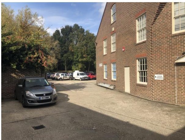
Figure 5: Existing access adjacent to Unit 3 (looking north).
