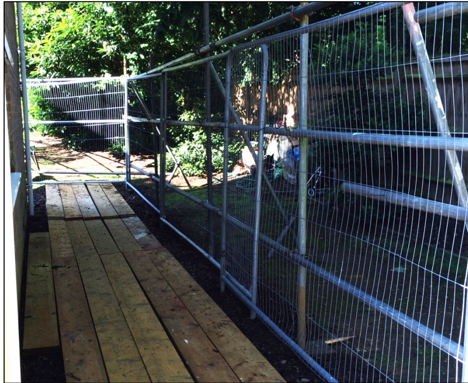
Scaffold board pedestrian ground protection
