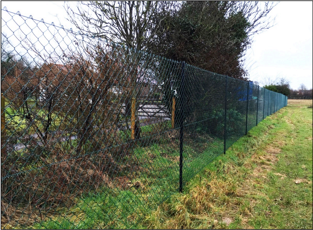
Chain-link on angle-iron uprights
