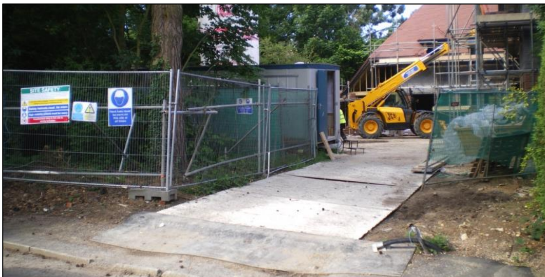
Vehicular ground protection trackway
