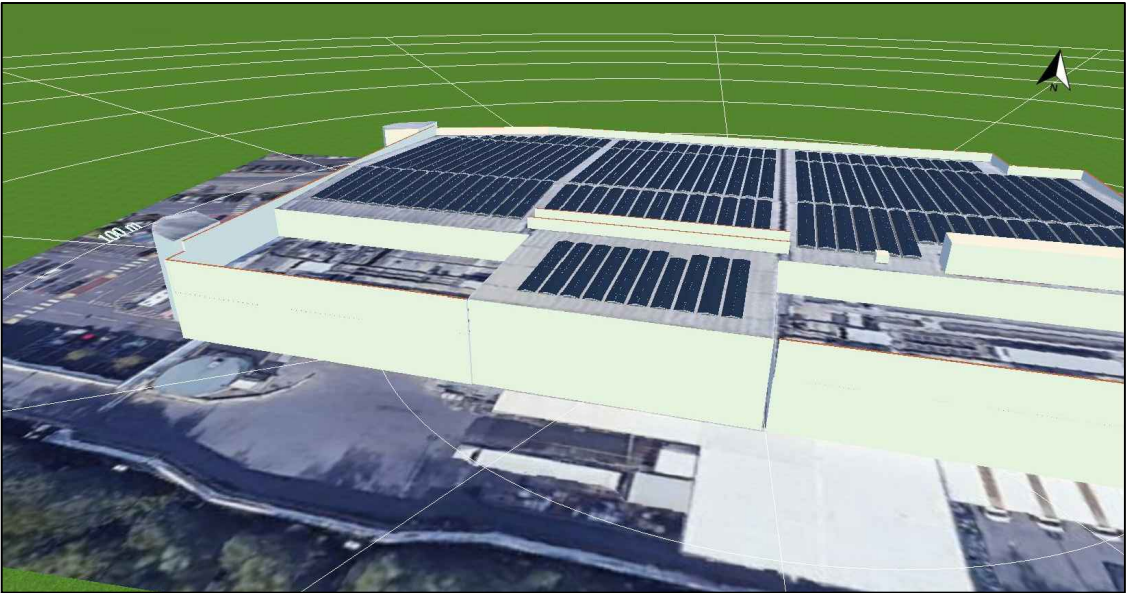
Existing Parapet Wall and Solar Photovoltaic Panels
