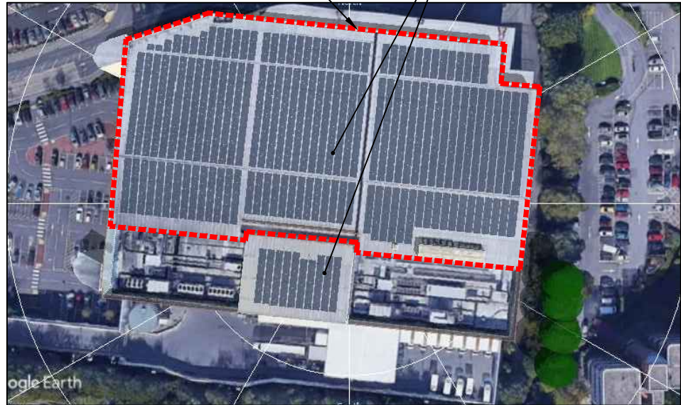
Existing Roof with Proposed Solar Photovoltaic Panels
