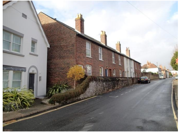
1. View from King Street
