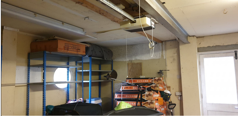
Figure 14. Internal view of the garage.
