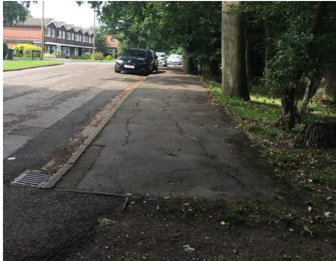
Photograph 4: Padnell Road - Northern Footway
