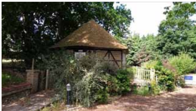
Photo 3. North-eastern elevation of Building 3
