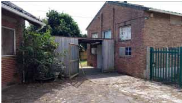
Photo 11. Northern elevation of Building 12
