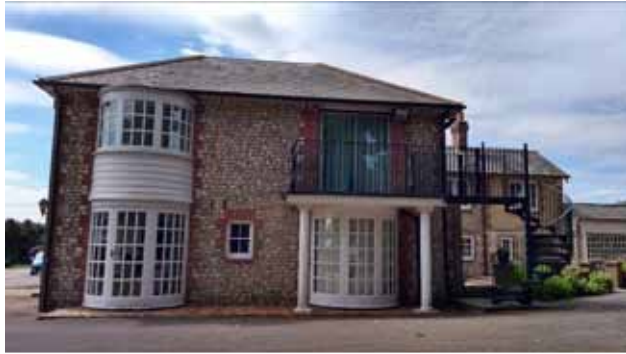
Photo 1. Eastern elevation of Building 1
