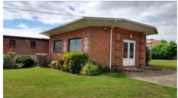
Photo 6. Northern and eastern elevations of Building 6
