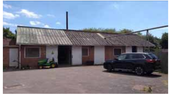
Photo 10. North-western elevation of Building 11
