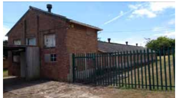
Photo 12. Eastern and northern elevations of Building 13
