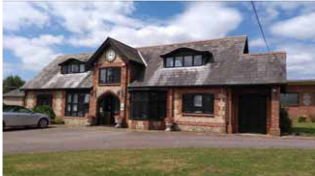
Photo 5. Eastern elevation of Building 5
