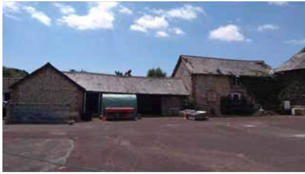
Photo 9. Northern elevation of Building 10
