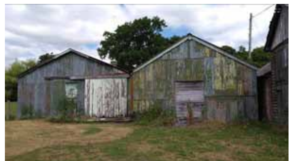
Photo 8. Southern elevations of Buildings 8 and 9
