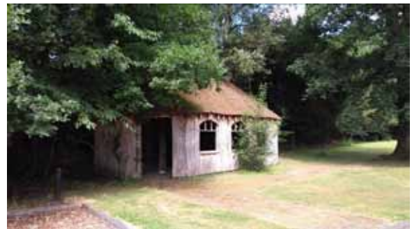
Photo 4. Eastern elevation of Building 4
