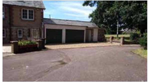
Photo 2. Northern elevation of Buildings 1 and 2
