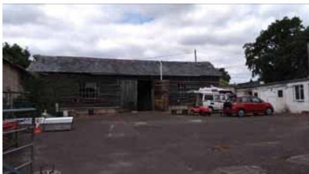
Photo 7. Eastern elevation of Building 7
