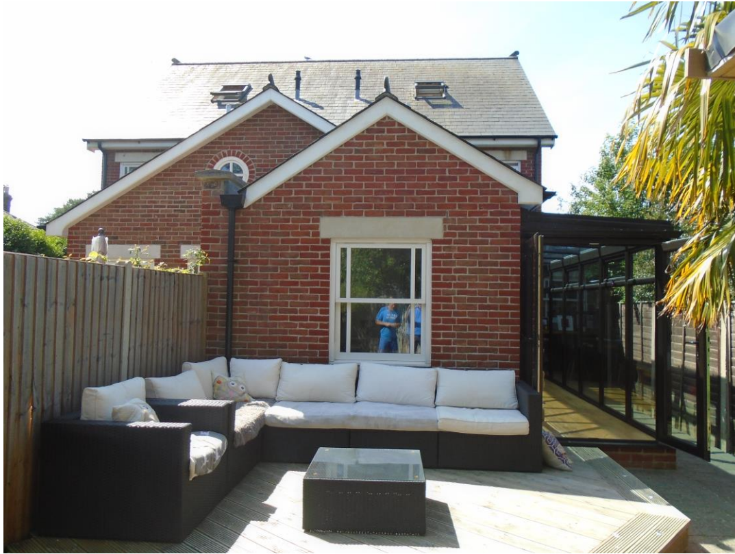
Figure 2. The rear of the dwelling.
