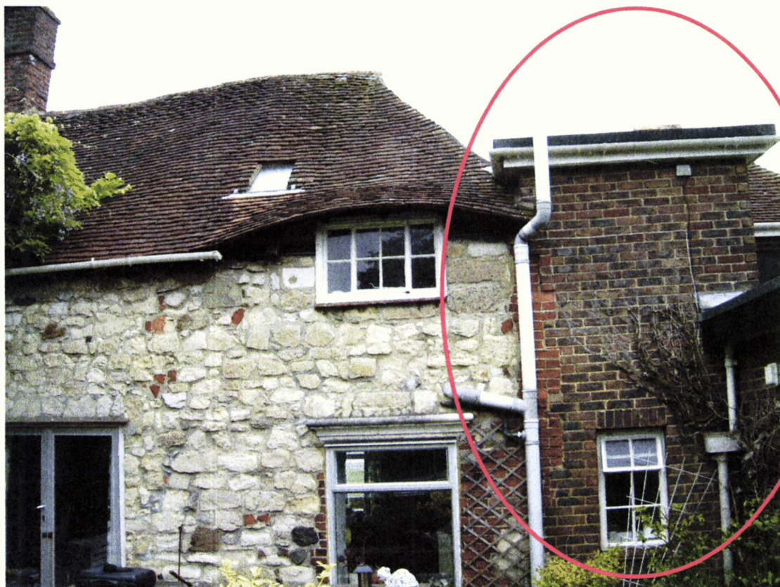
Part west elevation, two storey addition with flat roof.
