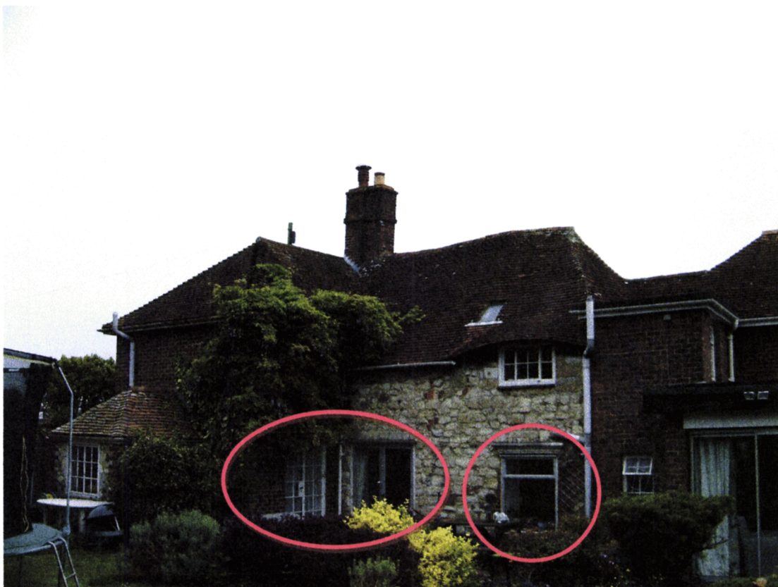
West facing aluminium window and doors, steel windows and doors.
