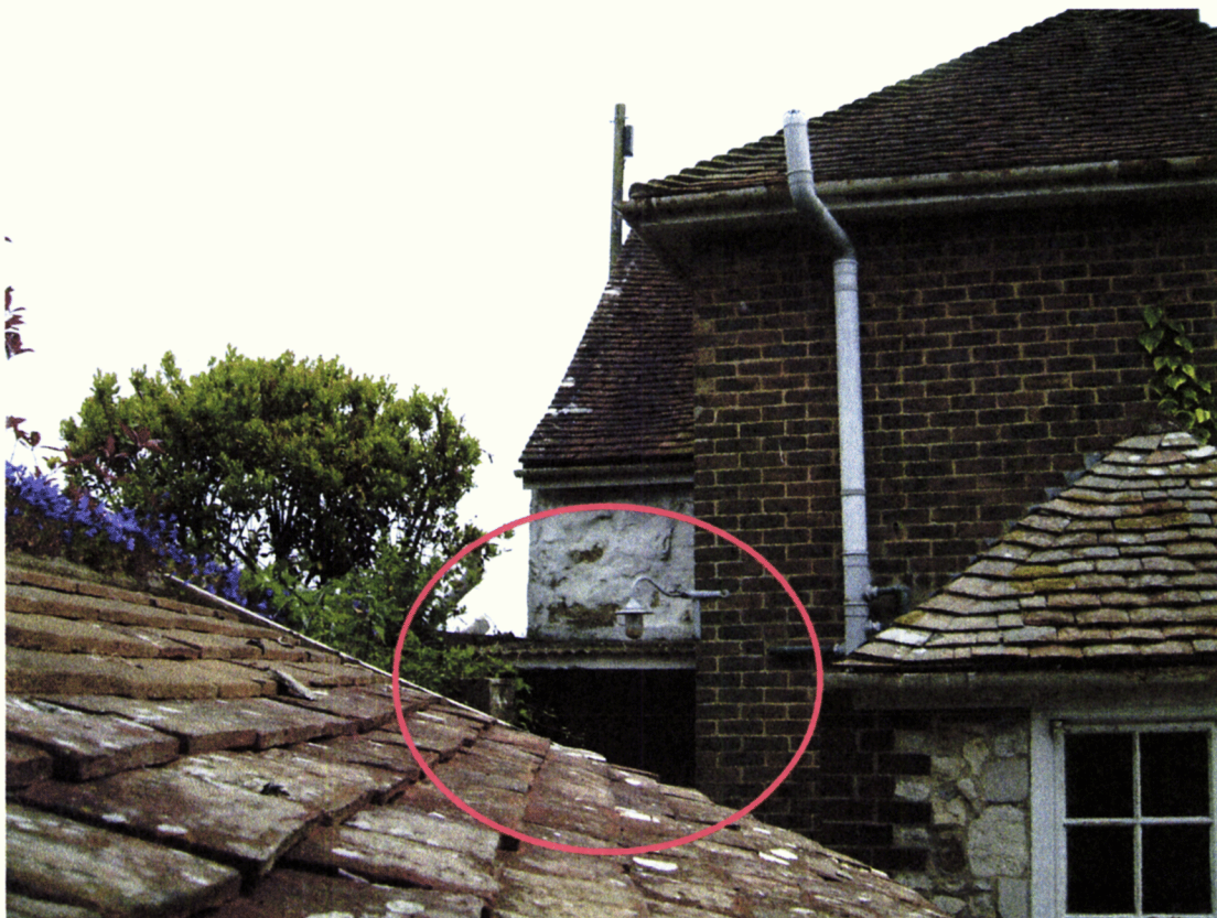
Corrugated roof structure attached to the dwelling and boundary wall.
