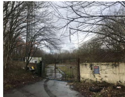
View of the gate at the entrance to the site with a tall mast just to the left of the entrance.
