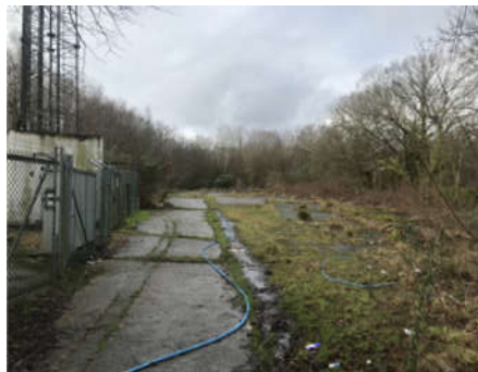
The concrete slab and overgrown greenery that covers the main area of the site.
