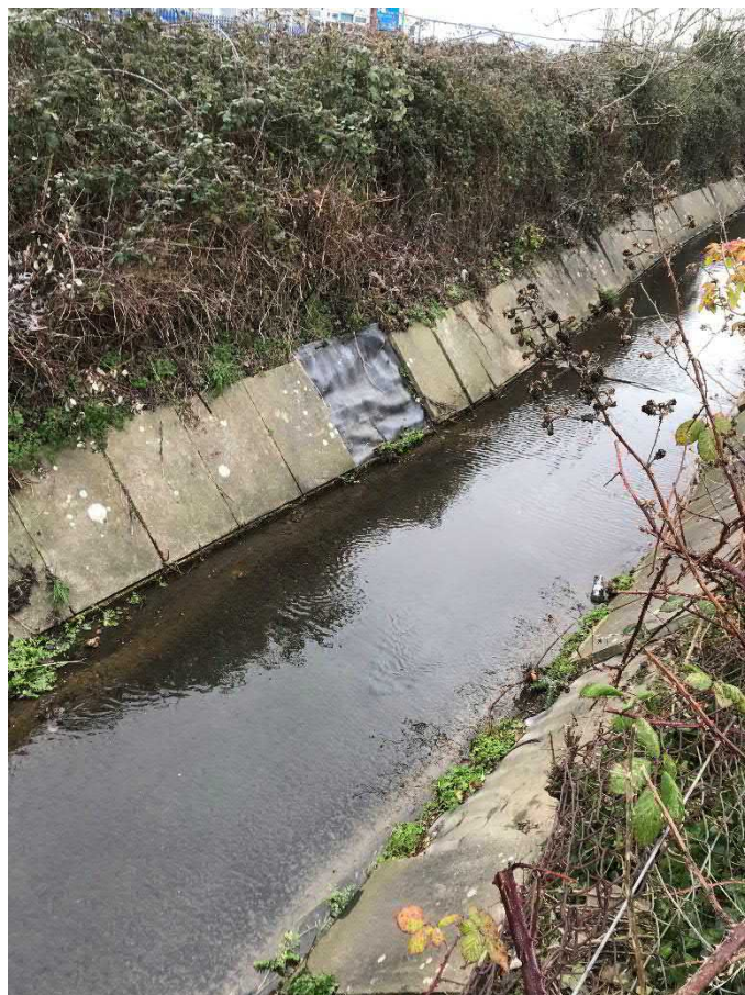
Image 4: Monsoon drain downstream of the outfall
