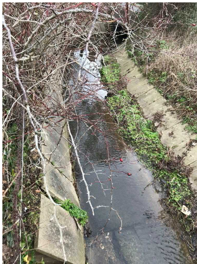
Image 2: River Lavant banks upstream of the outfall
