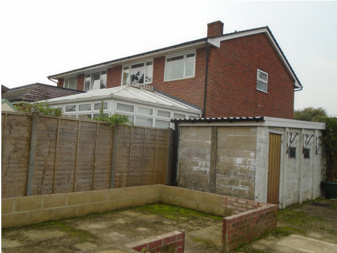
Figure 3. High fences enclose the application site at the rear.
