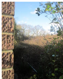
Vegetation to left hand side of property
