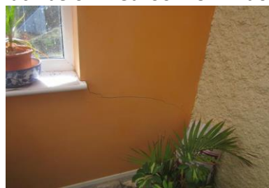
Right hand elevation - Tapering diagonal crack below Bedroom 3 window
