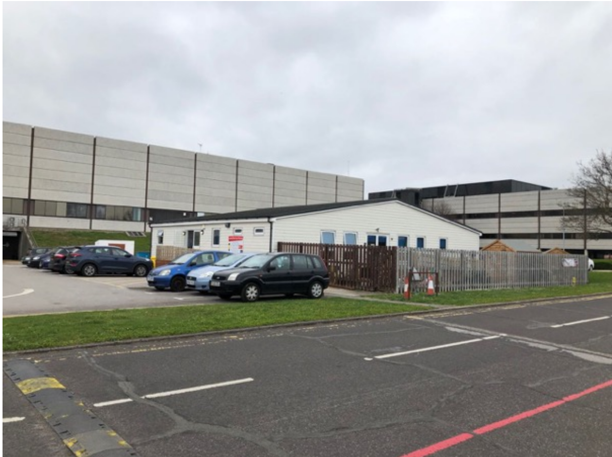
Figure 20. Building 5 (the nursery) which is clad with wood effect material and has a gable roof with tight fitting concrete tiles.
