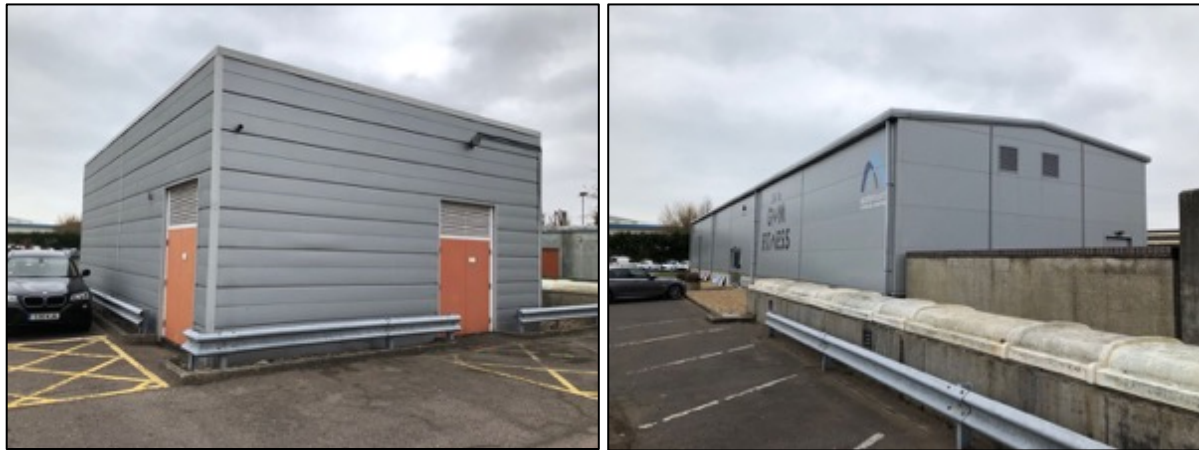
Figure 22. Left – Building 8. Right – Building 9 which is used as a gym.
