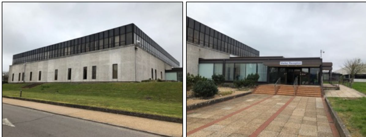
Figure 13. Left - Building 1 with vertical concrete cladding on the lower floor and glass panels on the upper floor. Right – The flat rooved extension on the northern face of Building 1.
