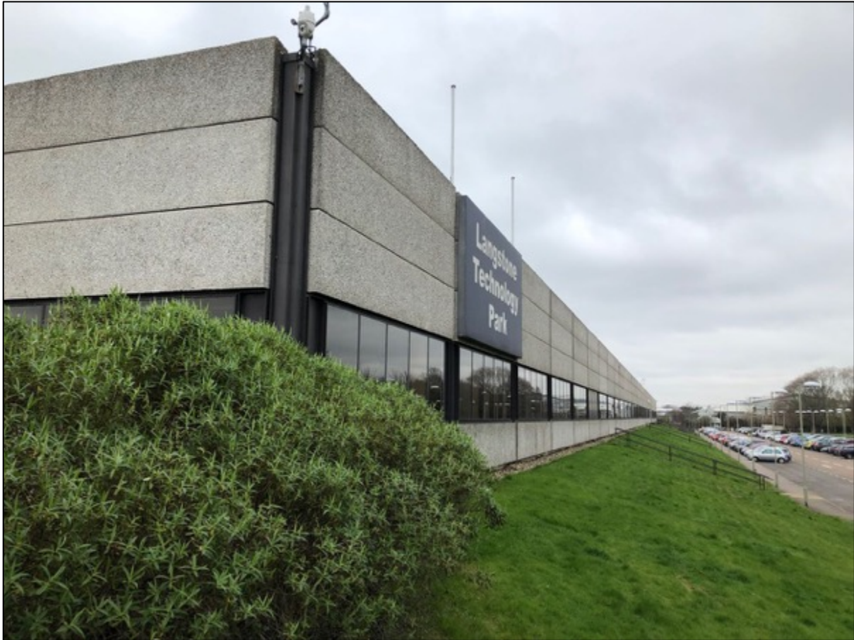
Figure 18. The northern elevation of Building 3, which is clad with horizontal concrete panels.
