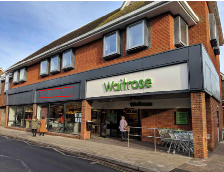
Current signage in-situ/Proposed signage location
