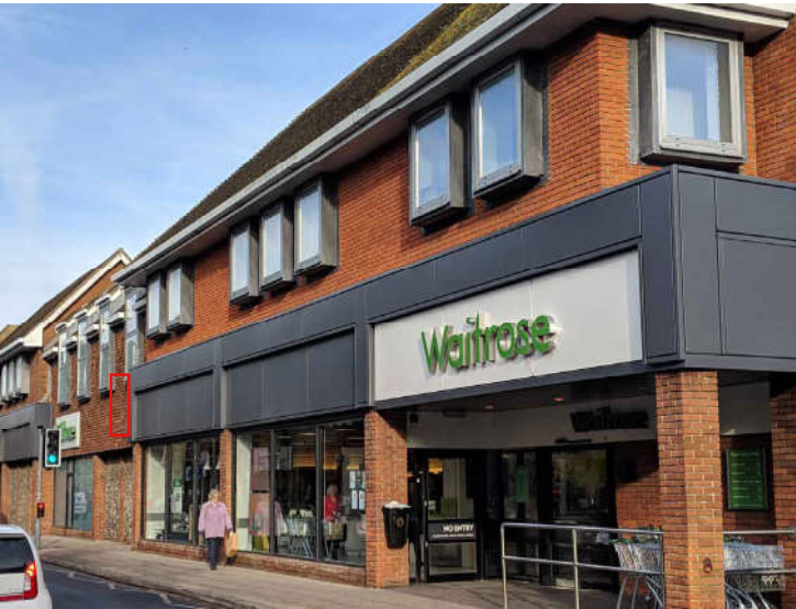
Current signage in-situ/Proposed signage location
