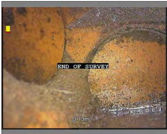
Photo: 008.JPG, VCR No.: 00005 3.13m, Manhole
