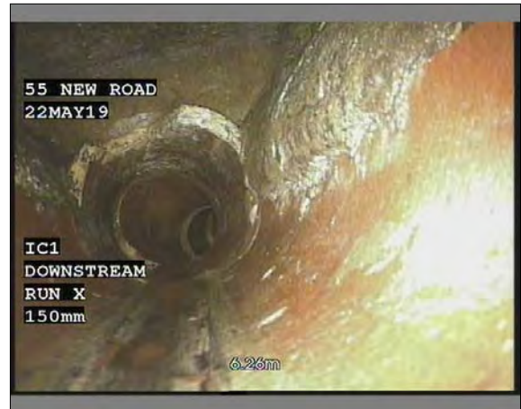
Photo: 007.JPG, VCR No.: 00004 6.26m, Manhole
