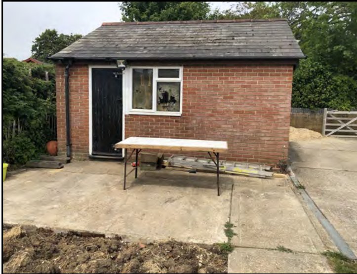
EXTENAL BUILDING UP THE FAR END OF THE GARDEN
