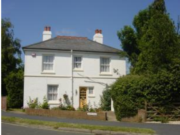
Figure 4: 23 Bath Road – prior to front extension. (2006)
