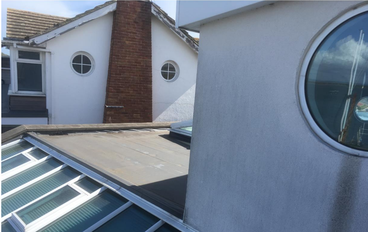
Figure 5 View from Rear Balcony of Spindrift towards West Elevation of Sinah House
