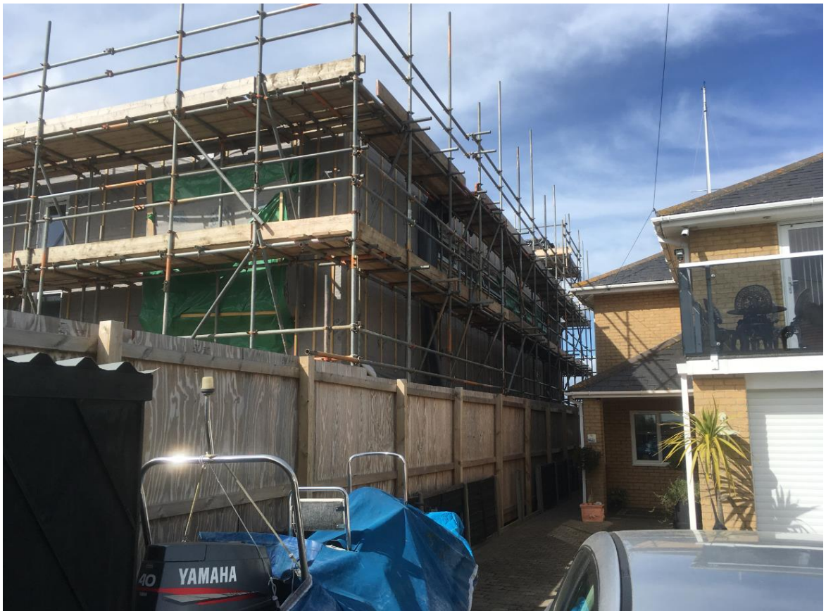
Figure 6 Relationship between “The Deck House” and Dwelling under Construction
