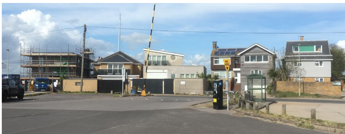
Figure 4 Streetscene Image of Row of Five Dwellings at Western End of Ferry Road
