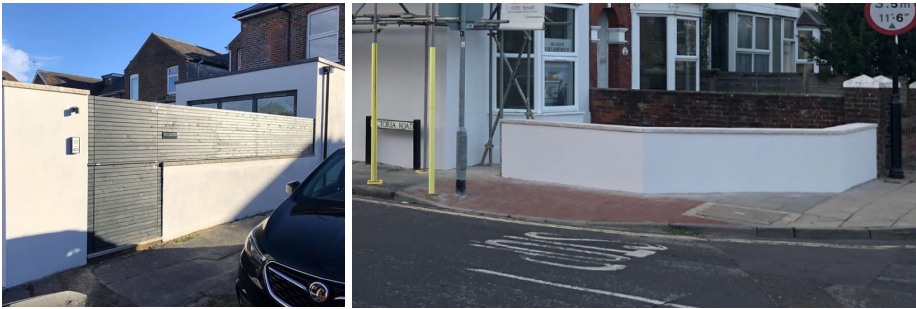
As completed rear and front wall photographs
