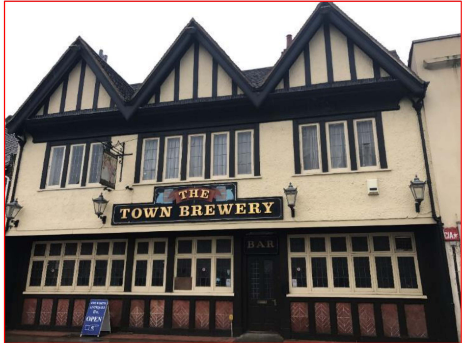
Plate 1 View of principal north facing elevation to the subject building.
