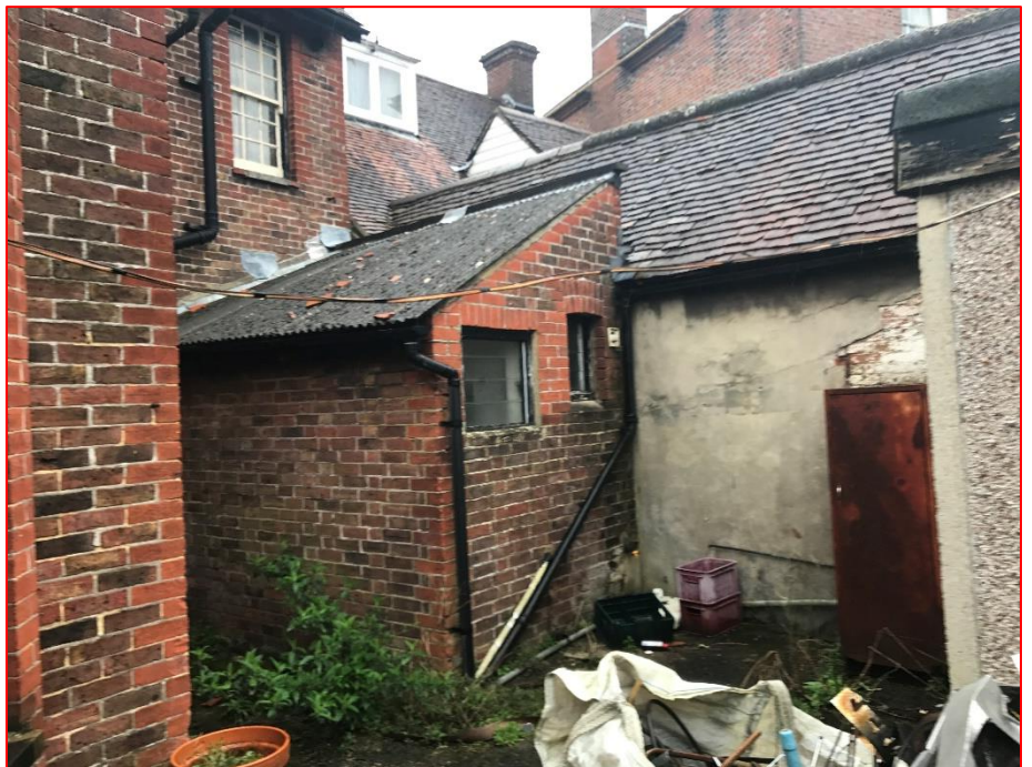
Plate 4 View of lean-to rear addition that adjoins the Grade II listed no. 1 High Street to the east.
