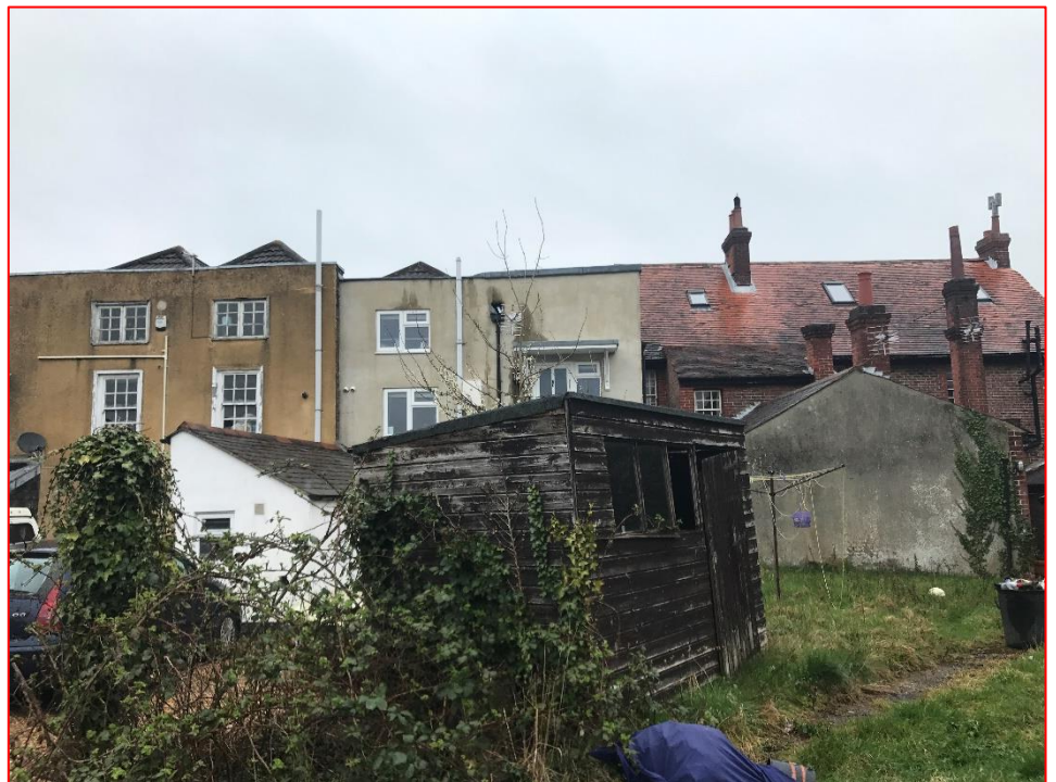
Plate 16 View of rear elevations to nos. 6, 8 and 10 West Street (centre and left of picture)
