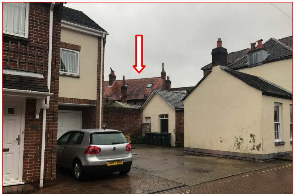
Plate 14 View of part of rear roof slope to subject building (arrowed) taken from School Lane. Note that the upper part of the two-storey addition will be partially visible in this view. Number 1F School Lane in the right of the picture, which is located to the rear of nos. 3, 3A and 5 High Street.
