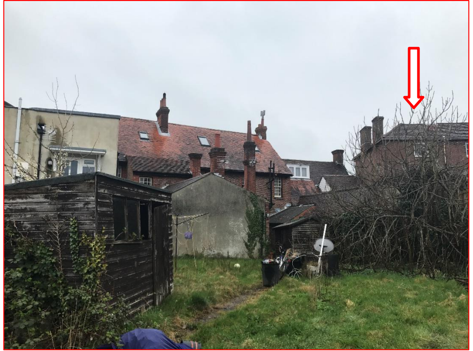
Plate 13 View of rear elevation to subject building (centre of picture). Note the Grade II listed nos. 3, 3A & 5 High Street (arrowed).
