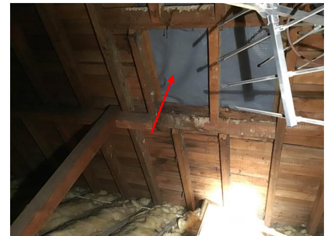
Plate 4.21: Exposed breathable membrane
