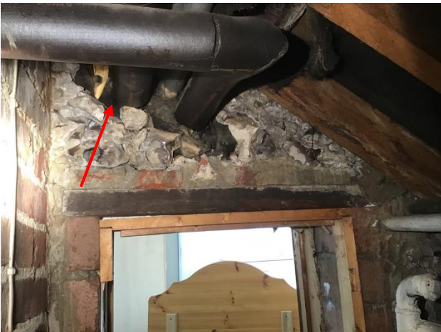
Plate 4.24: Damaged flint
