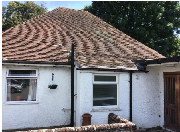
Plate 4.2: Single storey extensions
