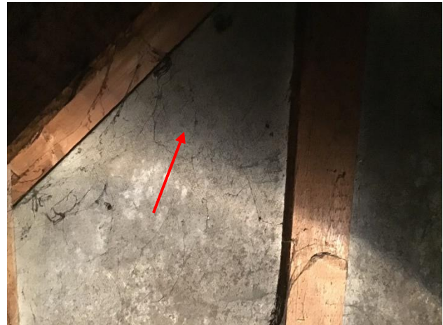
Plate 4.19: Asbestos board
