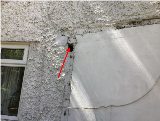
Plate 4.13: Gap in the wall where part of the building was demolished
