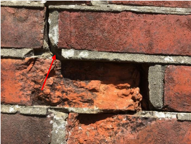
Plate 4.25: Damaged brickwork
