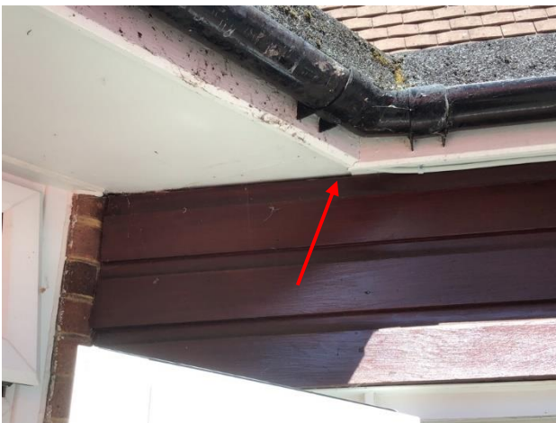
Plate 4.15: Gap between weatherboarding and roof
