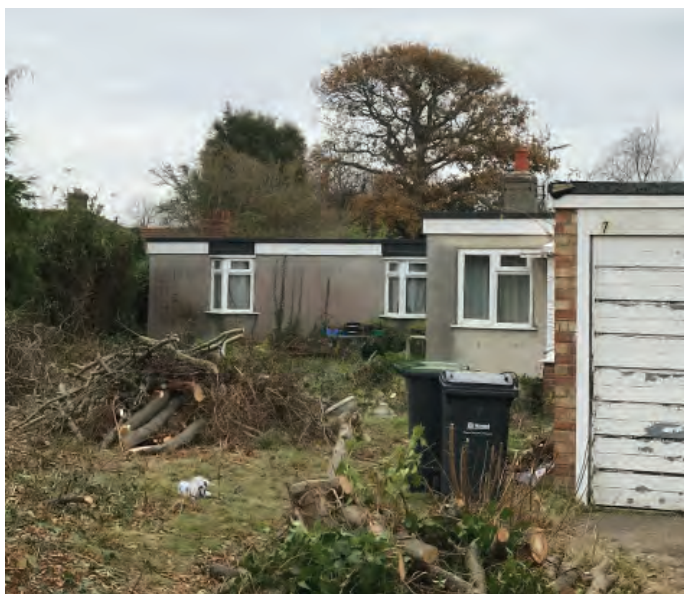
Existing dwelling at 7 Selsmore Avenue
