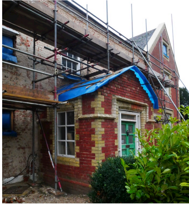
Exterior of Porch (November 2018). SW corner is parting from the main elevation.
