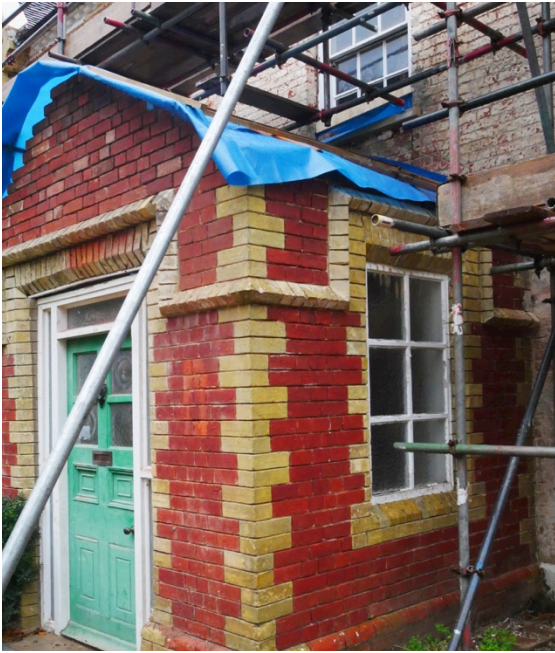
Exterior of Porch (November 2018). SW corner is parting from the main elevation.
