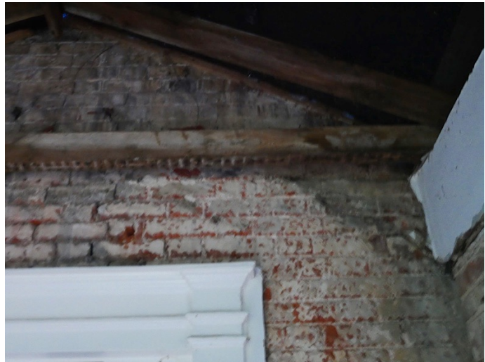
Interior: evidence of plaster finish and scar of previous smaller porch. Also evidence of damp and rot to end of rafters which require new sections spliced in with scarf repair.
