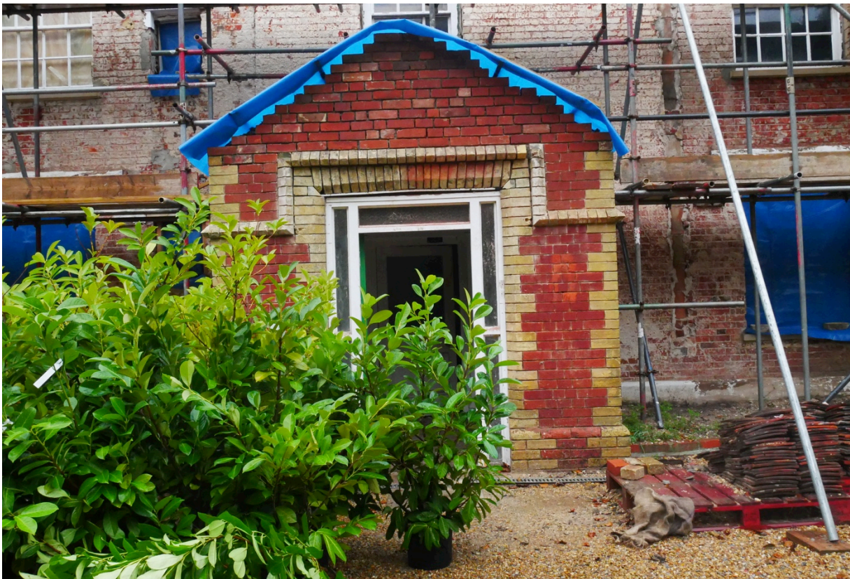
Tiles salvaged and stored on pallet for reuse (November 2018)
