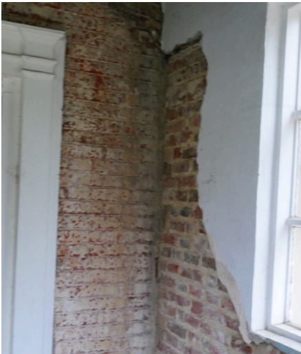
Interior: evidence of plaster finish and scar of previous smaller porch. Also evidence of damp and rot to end of rafters which require new sections spliced in with scarf repair.
