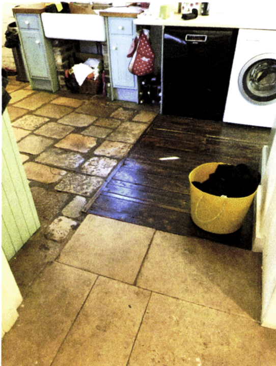
Fig.7 – Flooring to dining area and kitchen.
