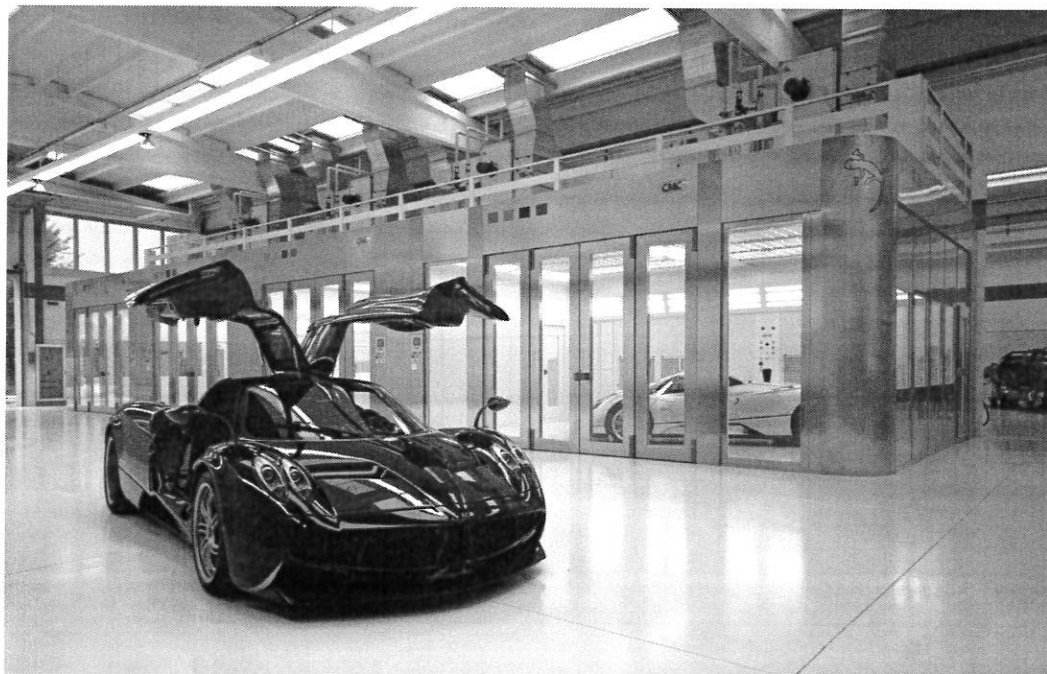
CMC spray booth and preparation equipment installed in the Pagani factory in Italy
