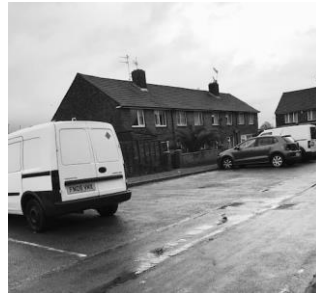
Photograph 31: Conditions During the Afternoon Survey (17.11.18)
