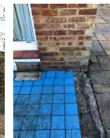
03/04 Existing paving in terrace area
