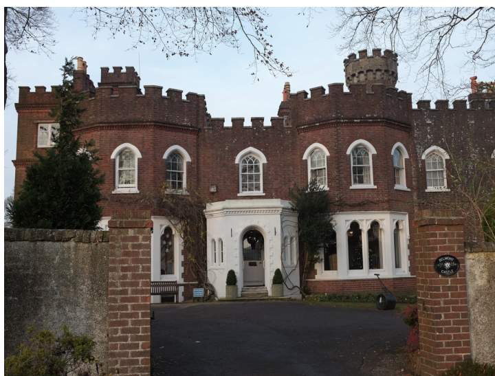
Plate 1 - Belmont Castle seen from Portsdown Hill Road
