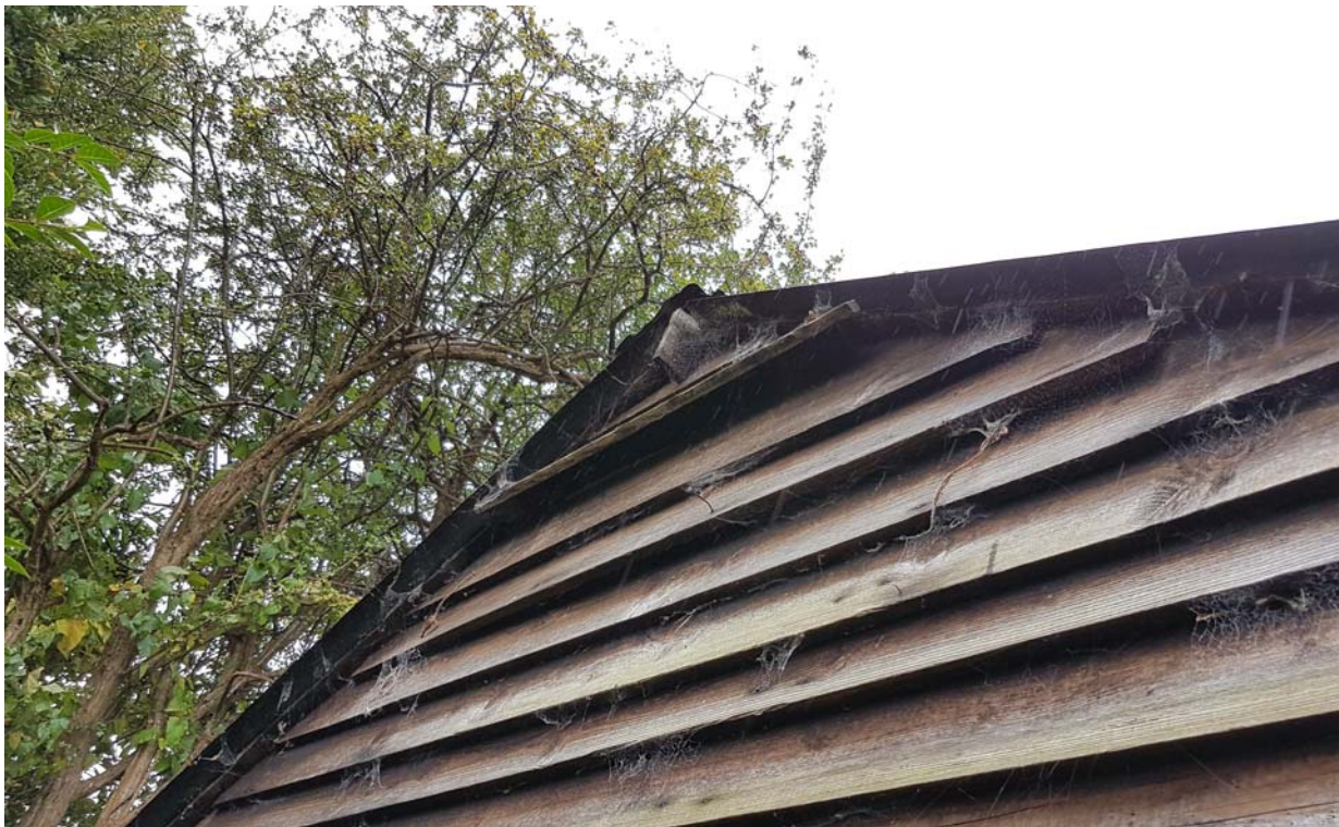
Photograph No. 06 - Purpose-made section of lifted weatherboard which could provide bird nesting opportunities. No evidence of bats was located.
