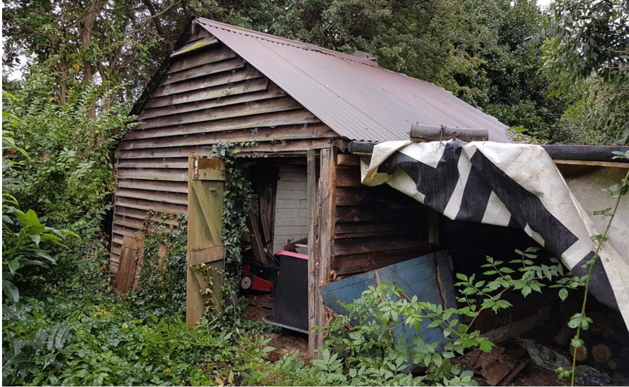
Photograph No. 05 - Small shed located to the south-eastern corner of the site.
