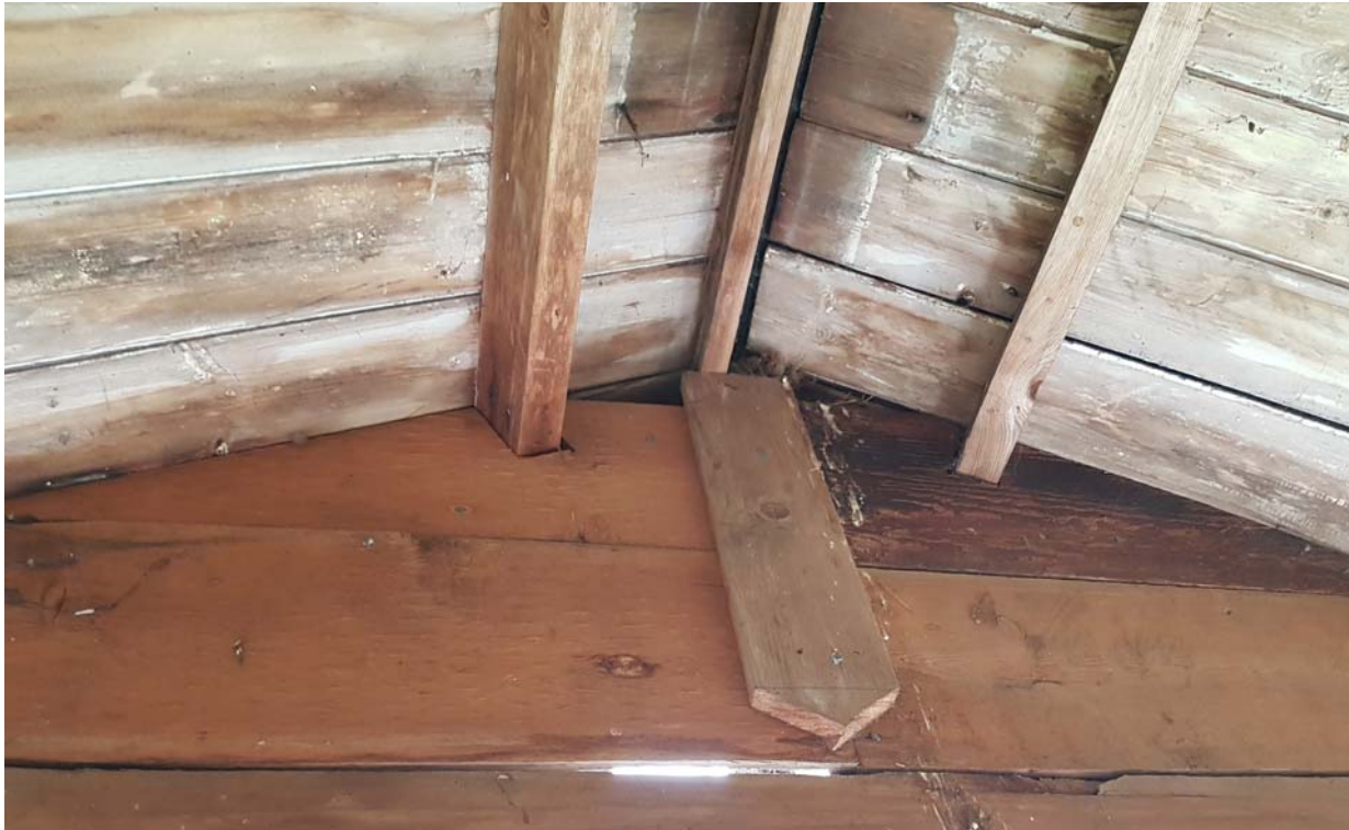
Photograph No. 09 - Small bird nest within the porch of the summer house.
