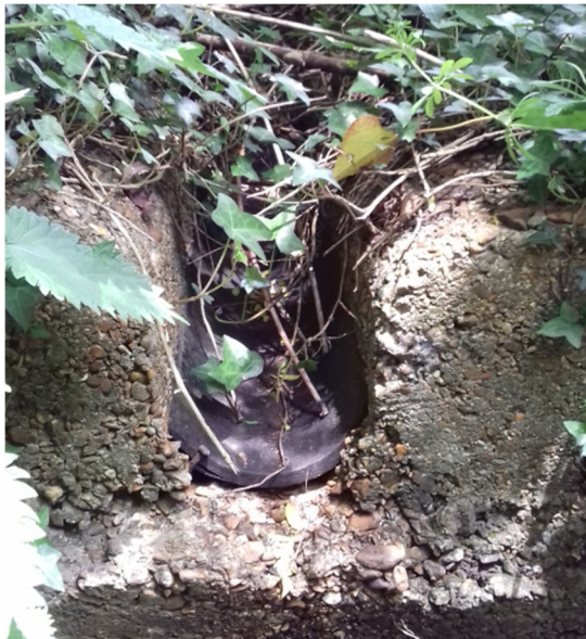
Figure 6: Existing outfall to Riders Stream
