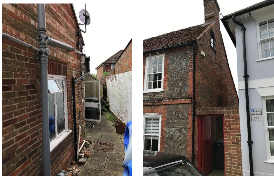
North West Elevation and Existing Side Access from King Street
