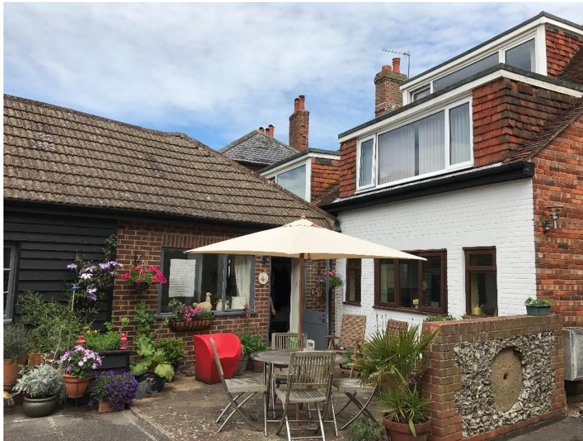
Existing Dormer, Low Flint Wall and Rear Elevation
