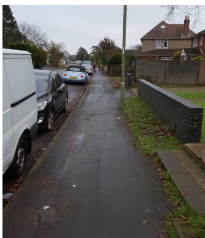
Photograph 7: St Mary's Road Footway
