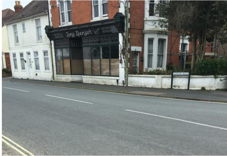
Photograph 2: Station Road Conditions
