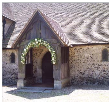
North door and timber porch
