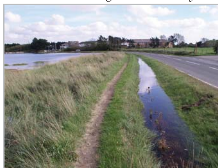
Flooded ditch at high tide, Northney Road
