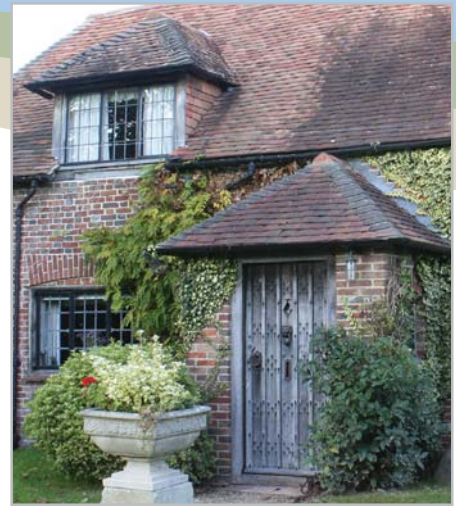
Porch at The Old House
