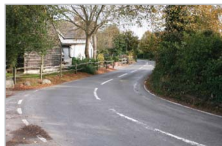
Sharp bend at Copse Lane
