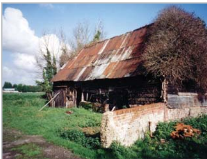
Brambles Barn before and after restoration in 2005
