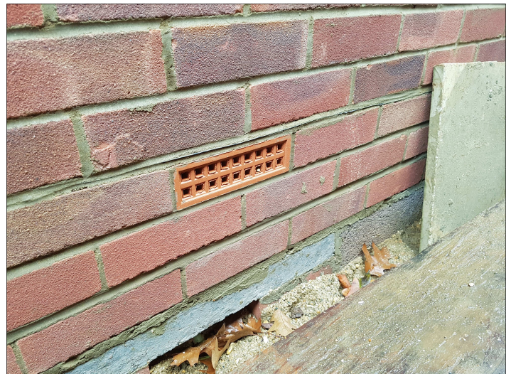
Steel reinforced concrete lintel over shallow drain
