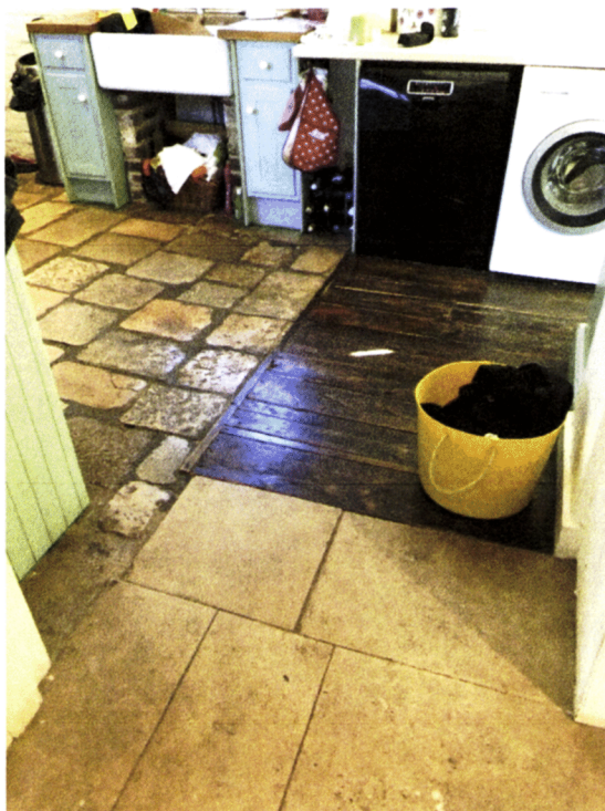
Fig.6 – Flooring to dining area and kitchen.
