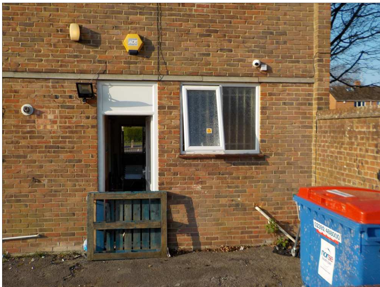
Rear of 39 Mill Road and location for newspaper secure storage unit and AC/refrigeration condensing unit
