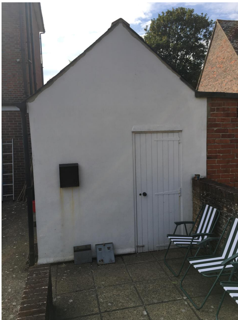
Existing Store Door
