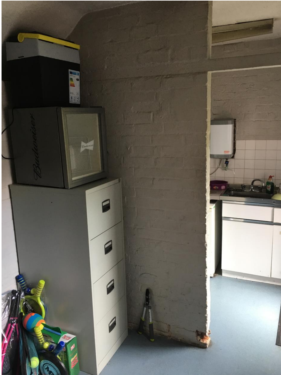
Internal Partition Wall
