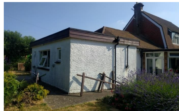
Figure 6 - The ancillary building to be demolished
