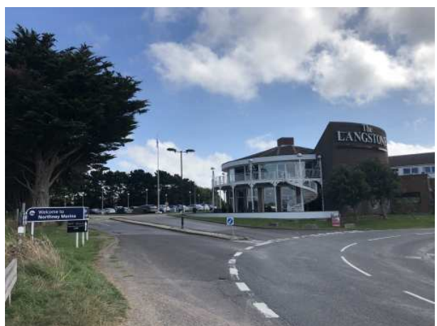
The approach to Langstone Quays from the west, on Northney Road.
