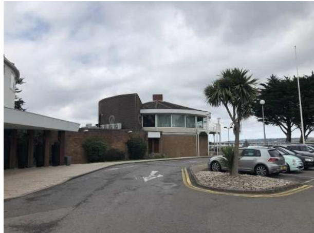
The application subject viewed from the east, on the frontage car park.
