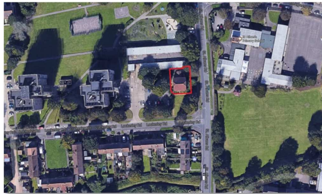
Fig 02: Aerial view of site [source: google maps]
