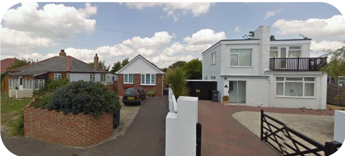
Existing Bungalow and Neighbouring Dwellings
