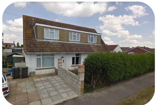
Large box dormer visible on front of chalet bungalow
