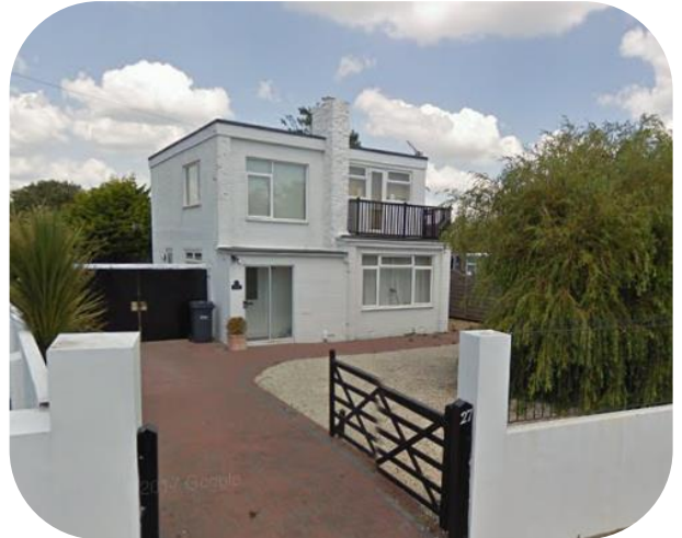
Neighbouring house consisting of a 2 storey flat roof built form
